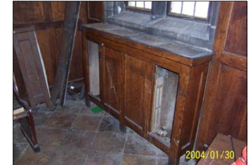
6 PHOTO RADIATOR ENCLOSURE TYPE A
