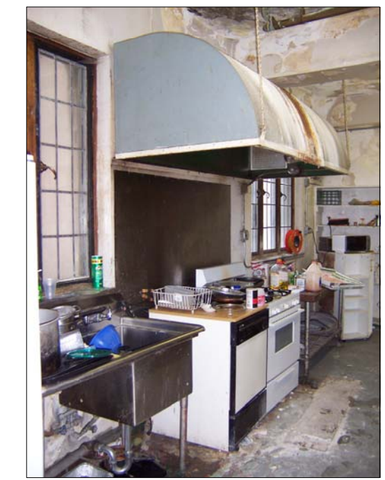
8 PHOTO KITCHEN LOOKING EAST
