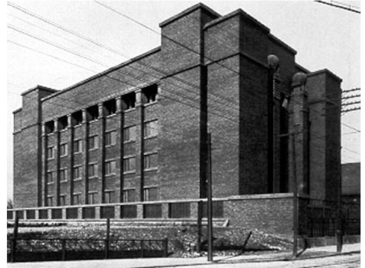
Larkin Building - Exterior
