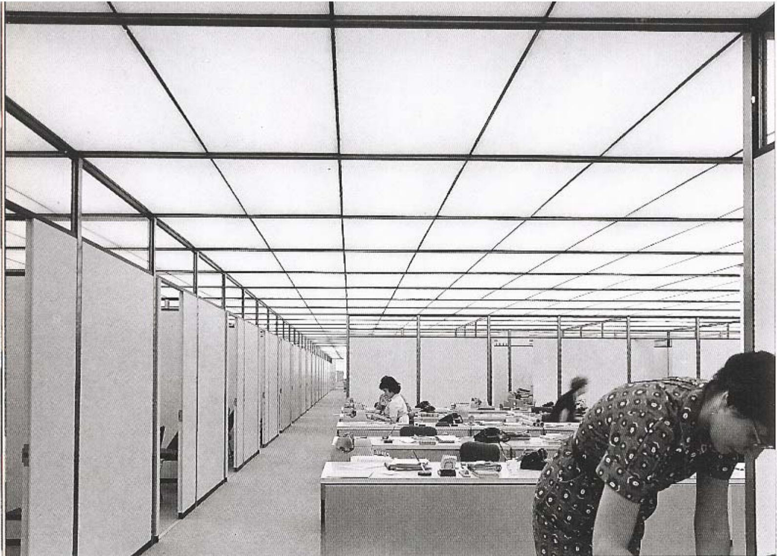
Gordon Bunshaft, Skidmore, Owings & Merrill (SOM) - Interior of the Connecticut General Life Insurance Company, Bloomfield, Connecticut, 1957
