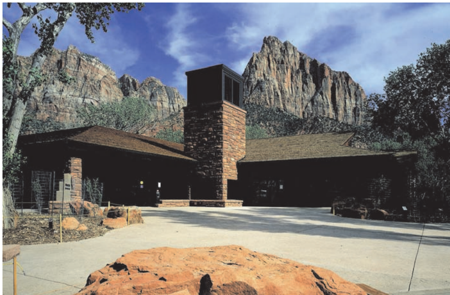
Figure 4-11. Zion National Park Visitor Center and Bookstore entryway showing the downdraft cooltowers and overhangs.
